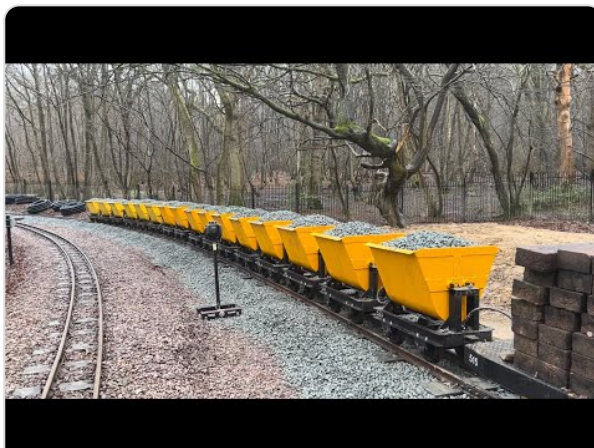
RUISLIP LIDO RAILWAY | BALLAST, BALLAST & MORE BALLAST
